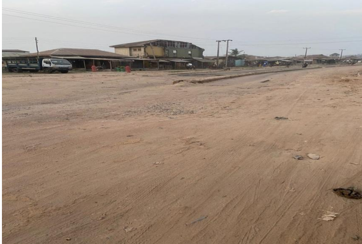
Plate 2: Abandoned Road Construction along Adatan. Source: Authors' Field Survey, 2024
