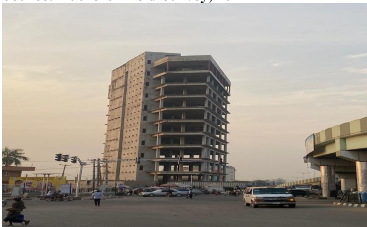
Plate 4: Abandoned Building Construction Project at Ita-Eko in Abeokuta. Source: Authors' Field Survey, 2024
