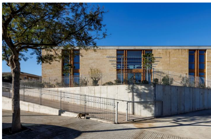
Figure 17: Ramp for access from street https://www.archdaily.com
