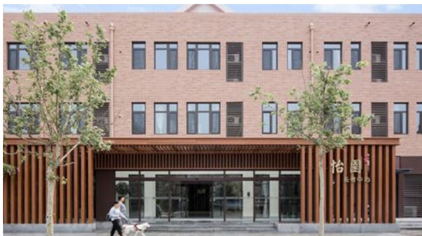
Figure 3: Front view of Yiyuan Service Centre for the Elderly
